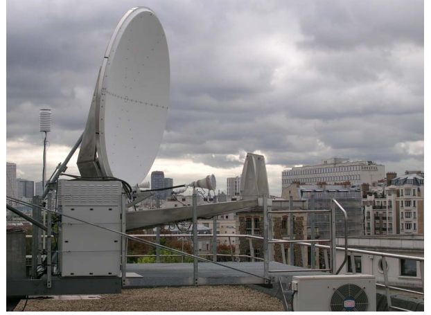
Figure 3. View of the two-way station and satellite simulator of LNE-SYRTE (Observatoire de Paris)
